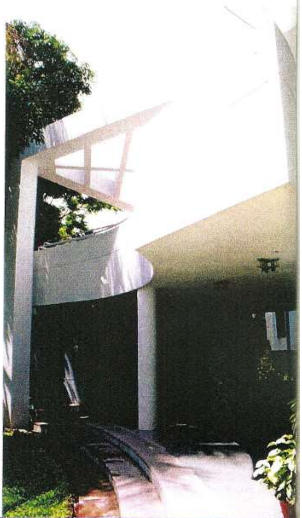
The covered verandah.
